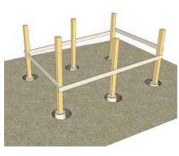
2. Pour concrete into sonotubes. Measure and cleat each post as shown above. Be sure to take the diagonal measurement before cleating in both directions. Back fill holes with gravel and let footings set for a couple of days before removing cleats.
