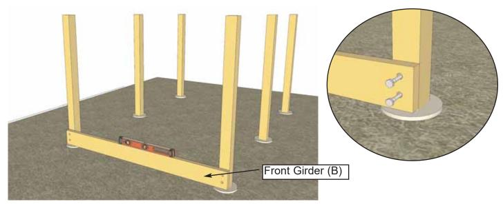
**3.** Once Posts have cured, locate a Front Girder (B) and position at bottom of front Posts. Make sure Girder is straight using a Level. Pilot hole Posts using 1/4" drill bit drilling through pre-drilled holes in Girder. Tighten Lag Screws (Washers) with 9/16" wrench. Complete all Lag Screws with Washers.
