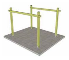
Lift, position and attach the second Post/Girder Assembly to Post Hardware.
