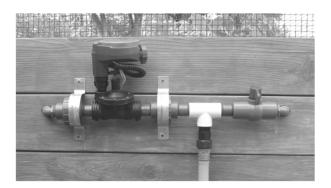
**Step 5 –** The long hose will feed through the other <sup>3</sup>/<sub>4</sub>" hole on the inside panel. Long hose may need to be cut shorter so it extends 1" past inside panel. Attach 90 degree elbow with hose nipple to each blue hose end on the inside. See picture below.
